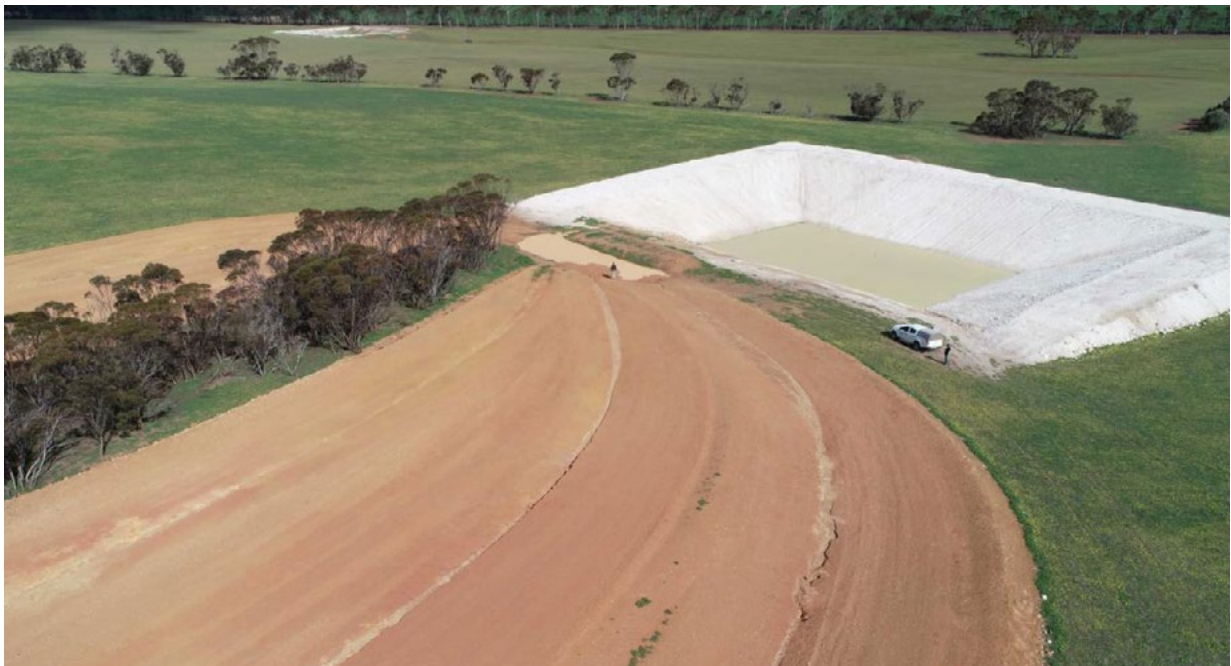
Roaded catchment can cause water to run after just 8–10mm of rainfall and with chemical treatment the threshold for runoff can be as low as 4–6mm. Source: South West Catchments Council
